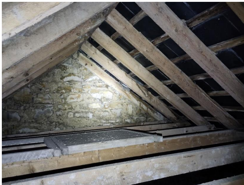
Figure 6: View of attic space.
