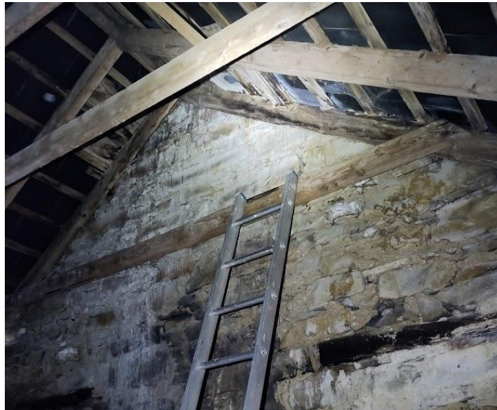
Figure 5: Ladder used to access attic space.
