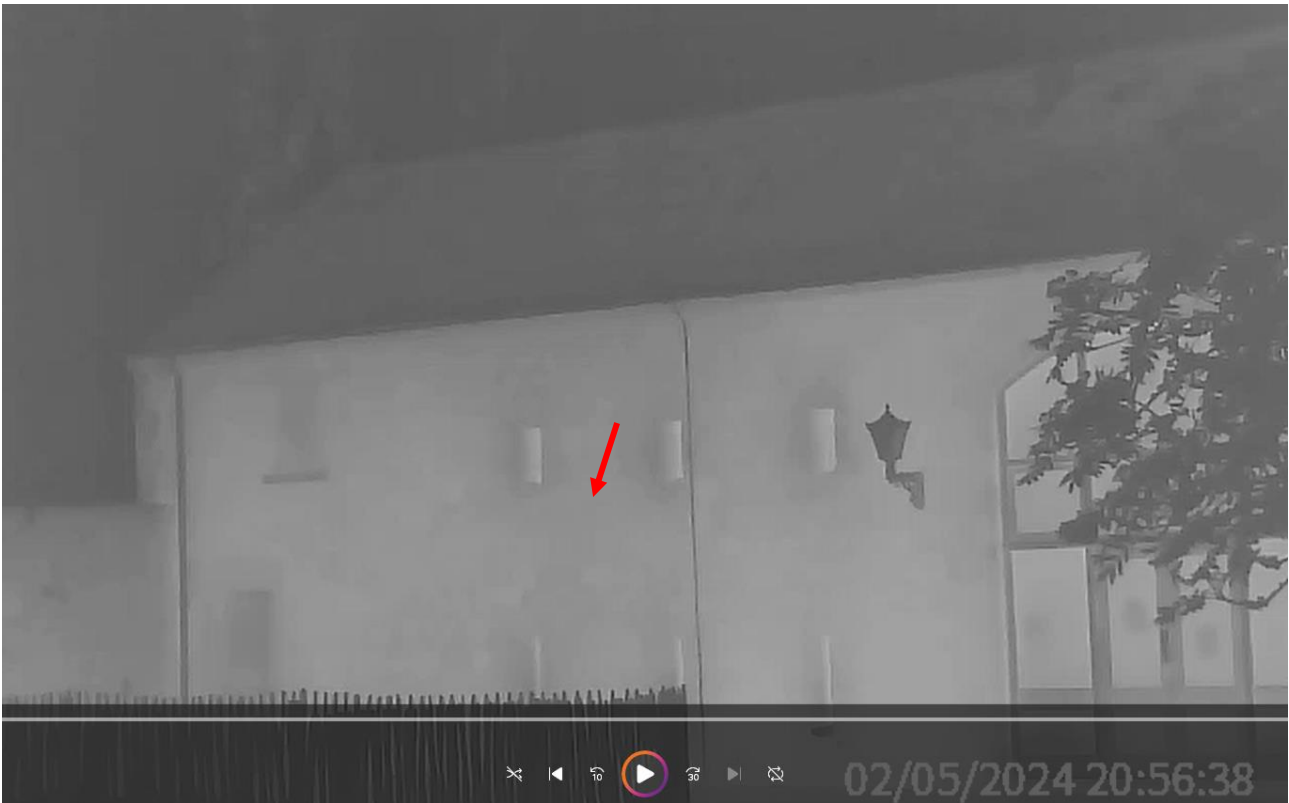
Plate 3: Screenshot of thermal image filming of rear of structure (red arrow – exit point for soprano pipistrelles).
