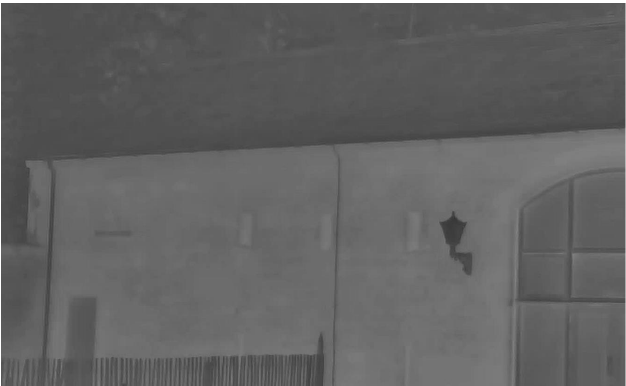
Plate 1: Screenshot of thermal image filming of rear of structure.
