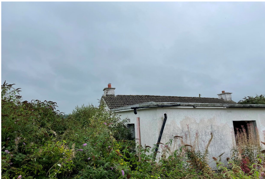
Plate 4-2: Confirmed maternity roost - flat roofed extension favoured by roosting pipistrelle bats.
