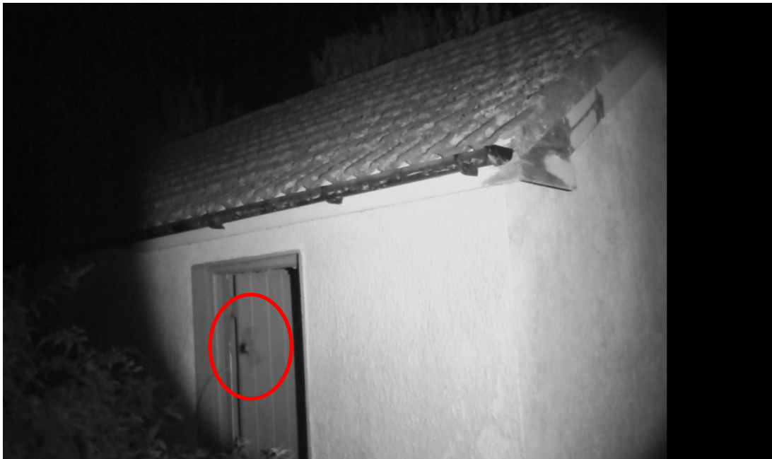
Plate 4-5: Bat access point – garage (structure 2)
