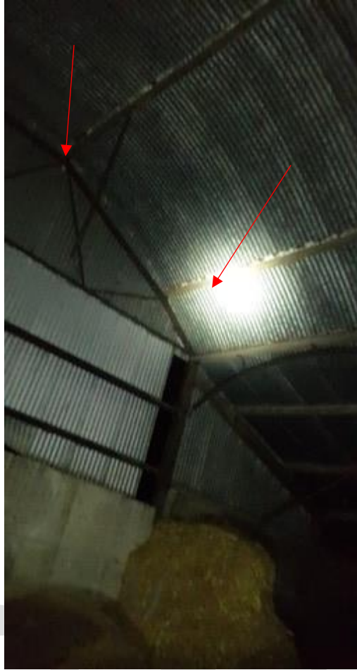
Roost areas in joists
