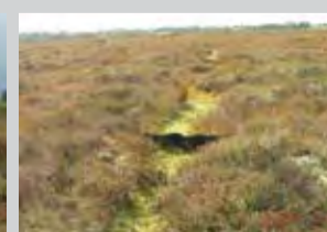
Drain blocking using plastic
