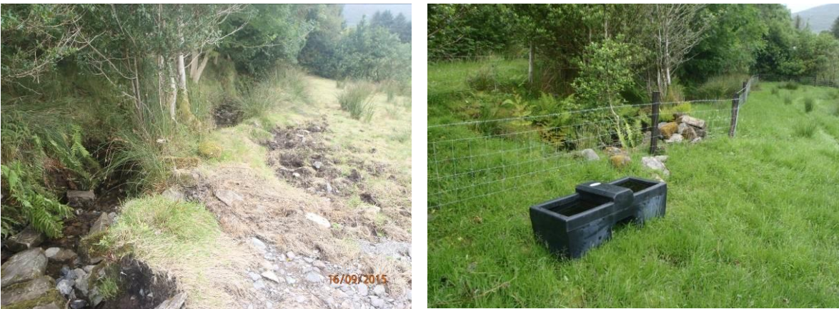
Figure 6 Example of drinking point before (September 2015) and after (September 2016) the fencing of the access point to the watercourse and the installation of a water trough.
